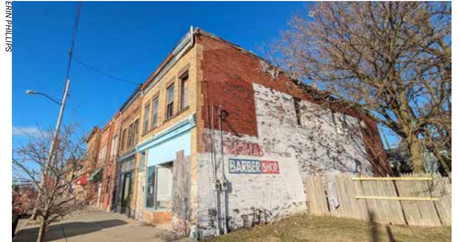
This corner at 13th and Parade streets is, according the HANDS CEO Matthew Good, "the only remaining source of blight in this section of Parade in Erie's East Side Midtown Neighborhood." It will soon be adaptively reused as affordable housing and will be dedicated as the "Emma Howell Apartments" in a partnership with historian Kevin Johnson and Preservation Erie.
