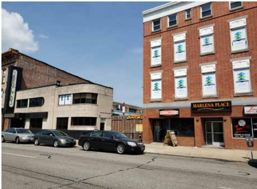
The Erie Downtown Development Corp. plans to transform the historic buildings it owns on Perry Square into a $30 million culinary district. The plans include demolishing the former Greyhound bus station and the building now known as Marlena's Place.
