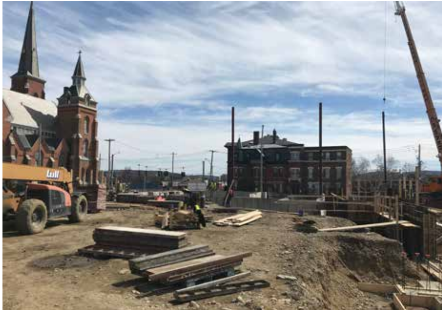
[left] Construction is underway on a $20 million, 49,000 square foot facility on the Elmira College campus that will serve as headquarters for LECOM at Elmira's osteopathic medicine program. [bottom right] An artist's rendering of the completed project, which will open its doors to 120 new medical students in July 2020.
